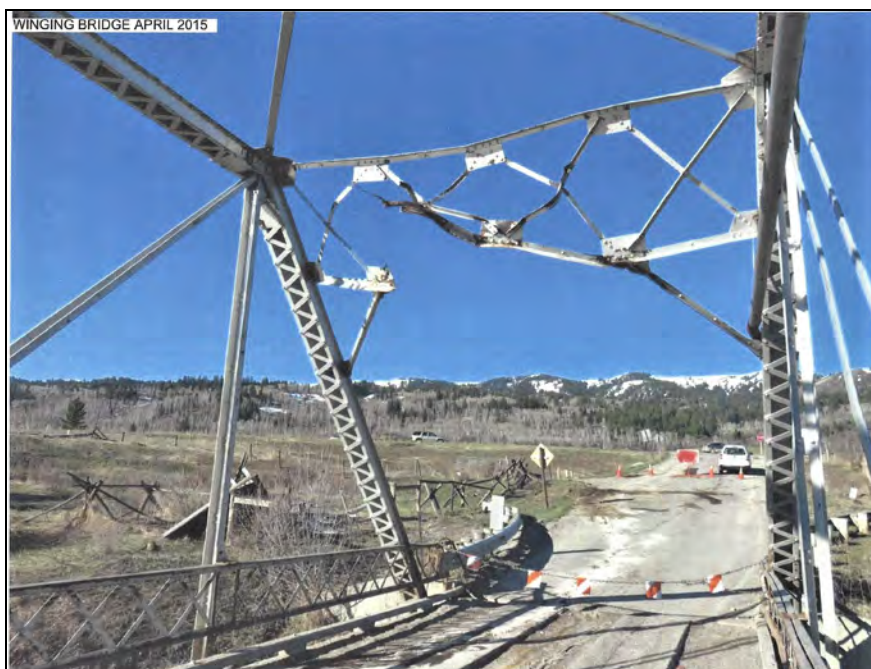
Figure 7. In April 2015, a large truck damaged the west span. It was repaired and opened for traffic in September 2015. (courtesy of Teton County Board of County Commissioners, Staff Report, 1/15/19)
